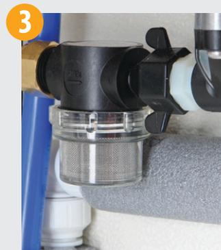
3 Check inline filter for any visual signs of leakage or damage to casing.
