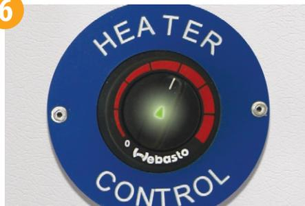
Finally, turn the heater control in the canteen clockwise to the "on" position; you should now see a solid green triangle in the centre of the heater control to show the heating is in working order.
