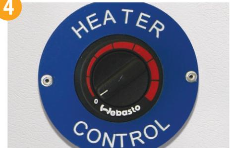
Return to the control panel in the canteen and turn heater control anti clockwise to the "off" position.
