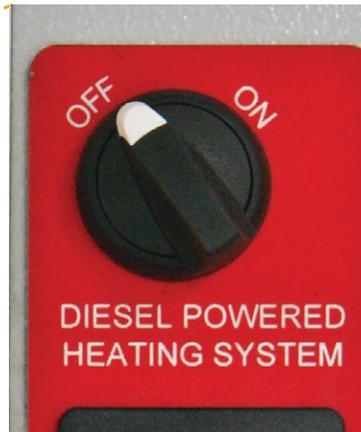
Turn the heater power isolator, situated on the 12V enclosure panel in the generator area, anticlockwise to the "OFF" position.
