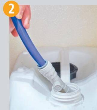
2 Ensure the non-return valve connected to the blue water pipe in the water butt is present.
